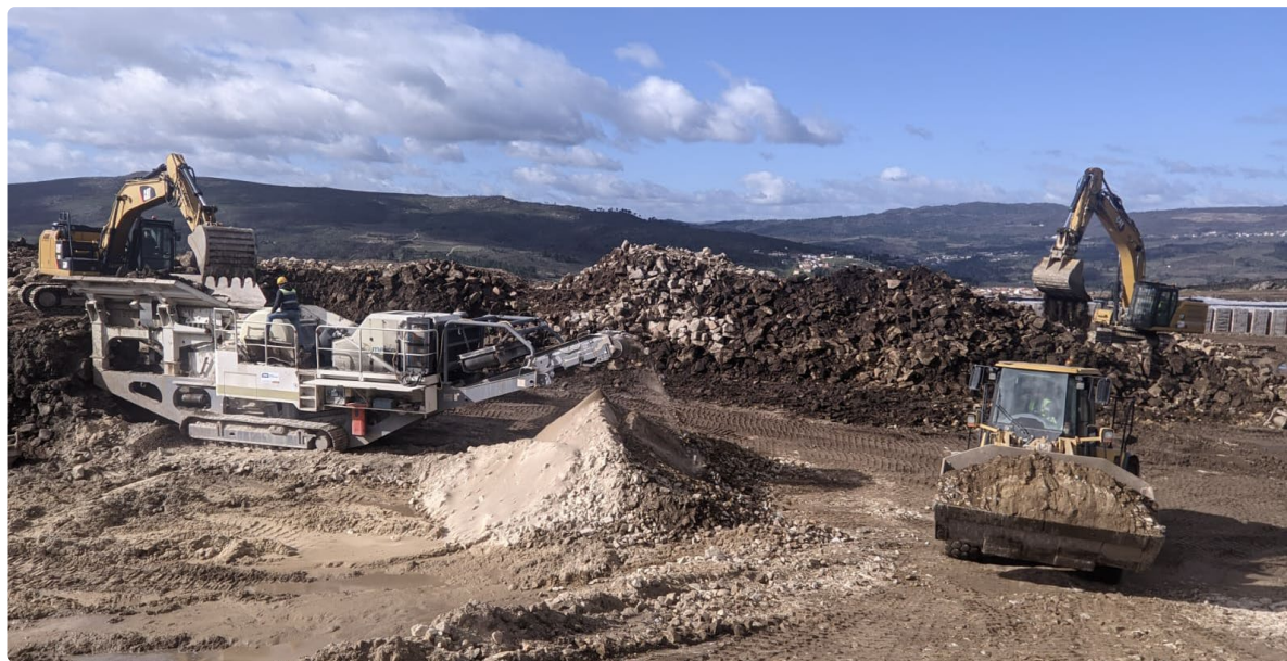
7 Figure 13: Riodades Solar Photovoltaic Park | Portugal
