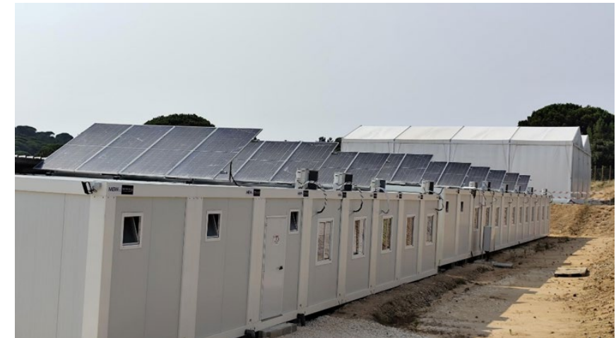
Figure 10: Cibeles Solar Photovoltaic Park | Portugal
