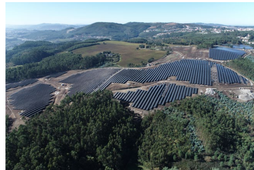
Figure 3: Felgueiras Solar Photovoltaic Park + BESS | Portugal
