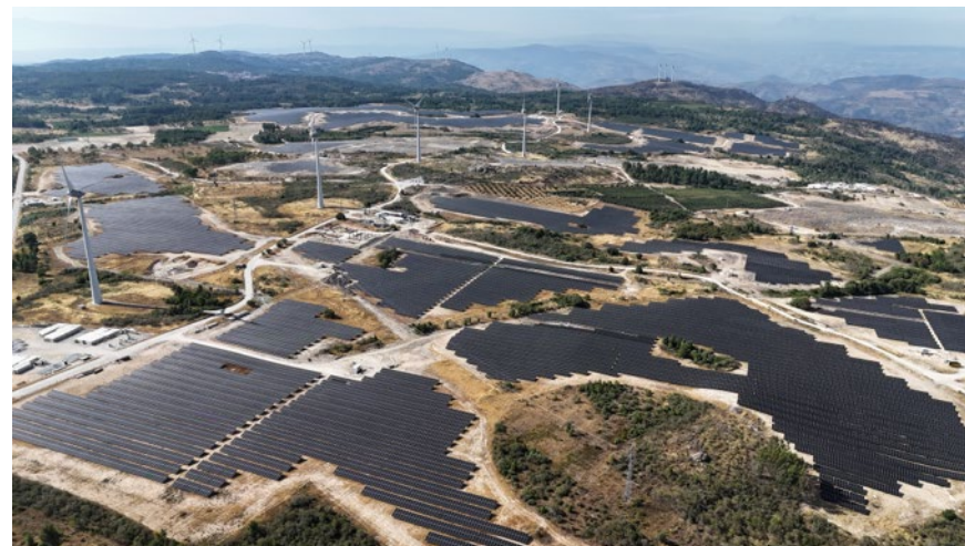
Figure 2: Sendim Solar Photovoltaic Park | Portugal
