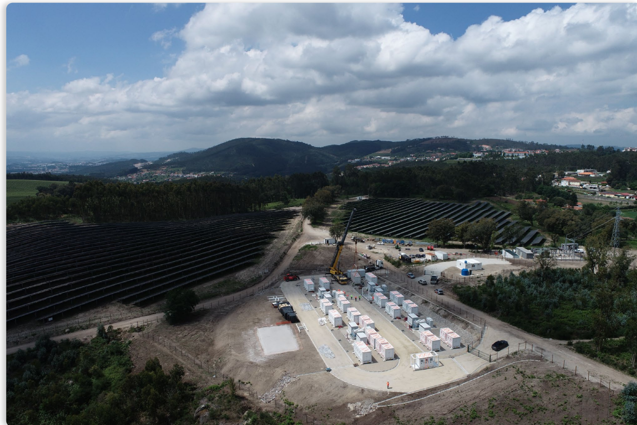
Figure 15: Felgueiras Solar Photovoltaic Park + BESS | Portugal
